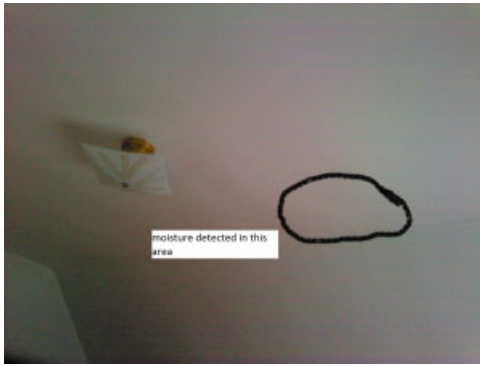
Moisture detected in the area where the flat ceiling meet the sloped surface
