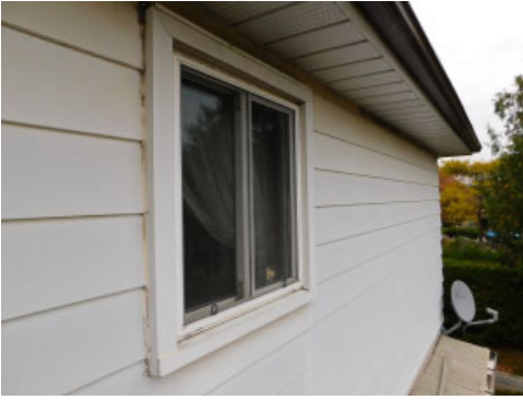
Upgrade caulking around all windows
