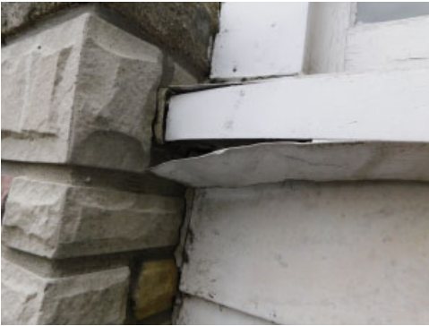
Upgrade caulking throughout - on front sunroom
