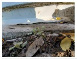
Front porch re caulking of flashing between slab and foundatioin wall is required
