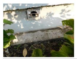
Recaulk flashing-Front porch- possible source of moisture on drywall in ceiling of storage area in bsmt
