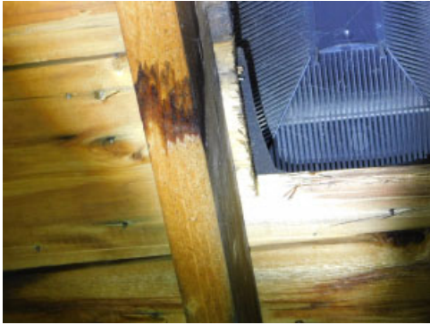
Wet rafter beside roof vent
