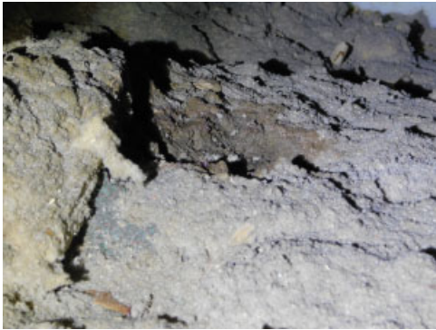
Wet insulation below roof vent. Have a roofing contractor inspect to determine cause
