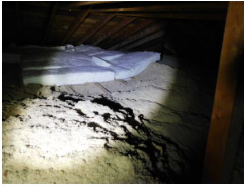
Unevenly installed insulation in the attic
