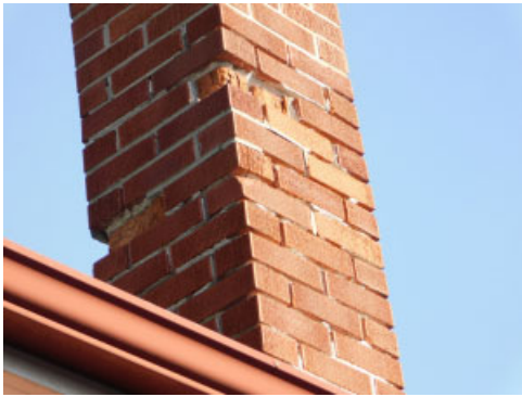
Chimney requires brick repairs. As it is obsolete it can also be removed
