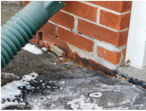
Tuck pointing and brick is required on the bottom courses of bricks adjacent to the garage door
