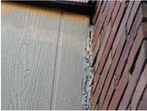
Upgrade caulking at front and rear sunrooms, between cladding and bricks.
