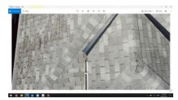
shingles on south side of roof is worn - expect to replace within 2 years
