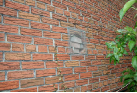
Repair hole for old exhaust vent on north wall
