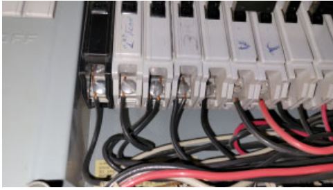
Double tapping of circuits on main panel
