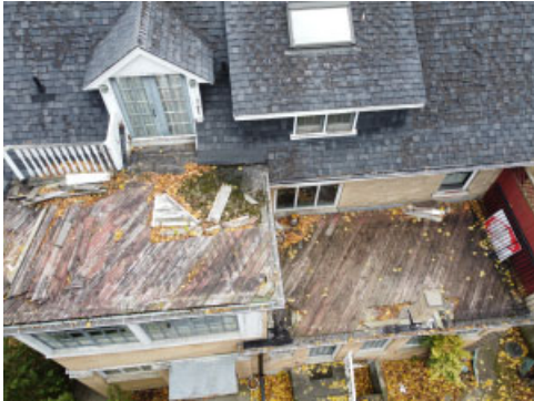
Tar and gravel roof under decking has to be replaced
