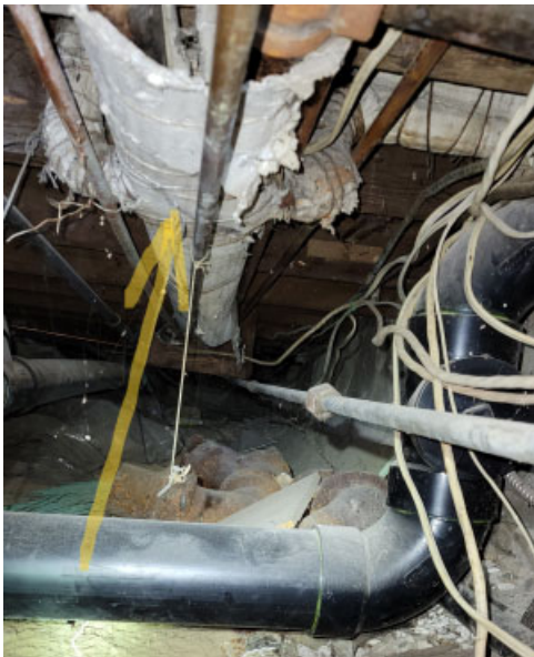
Asbestos wrap on heating pipes in crawlspace
