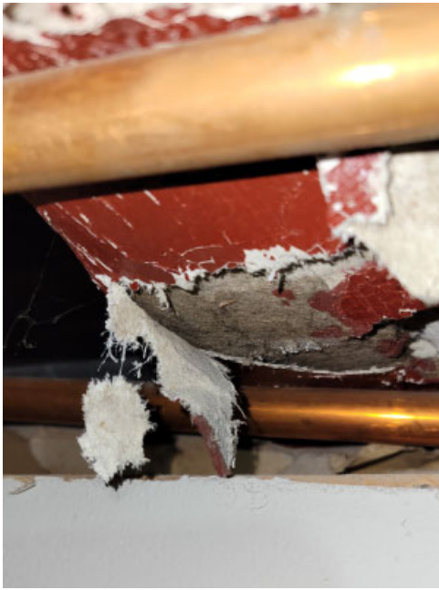
Asbestos wrap on heating pipes above the boiler
