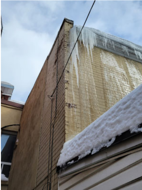
Excessive ice build up on getters and wall - Indicates insufficient insulation in the flat roof cavity
