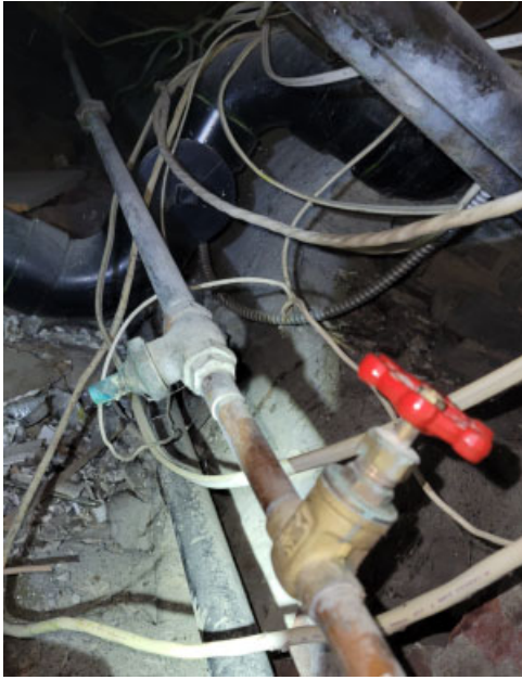
Galvanized steel water supply line in the crawlspace
