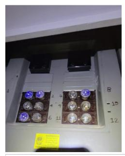
Fuse panel should be upgraded to a breaker panel
