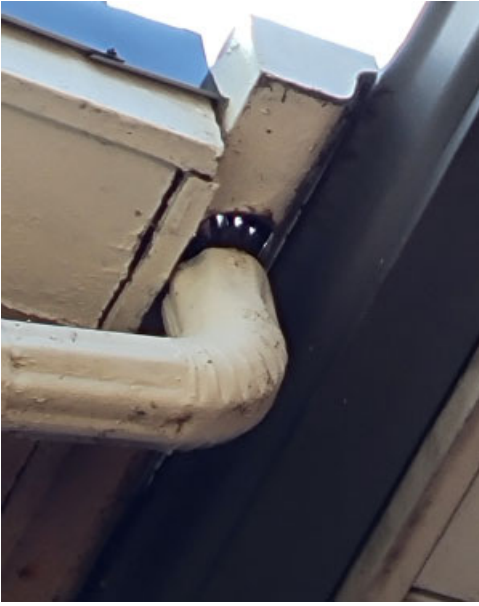
gutter is not connected to the downspout
