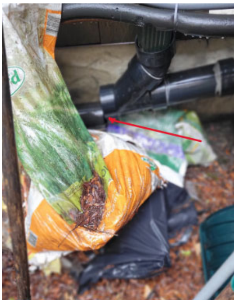
Discharge pipe connected to the downspout is disconnected. Water is discharging against foundation.
