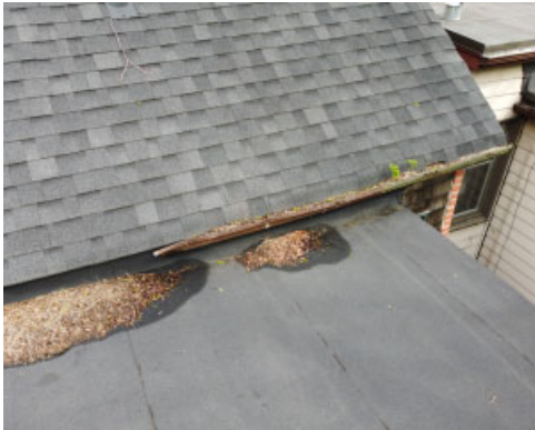
Seasonal cleaning of gutters and debris on flat roof is recommended
