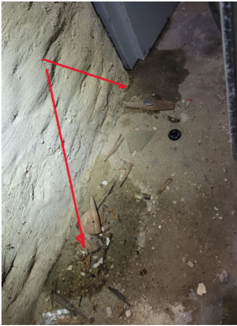
Active leak. Corresponds to location of disconnected downspout on the exterior
