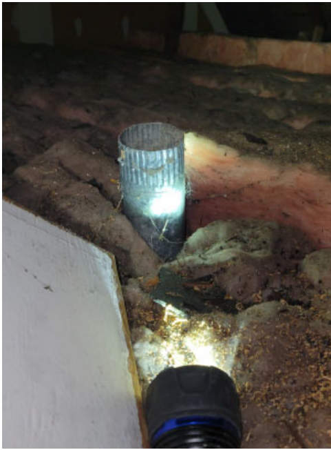
Washroom exhaust vent terminates in the attic
