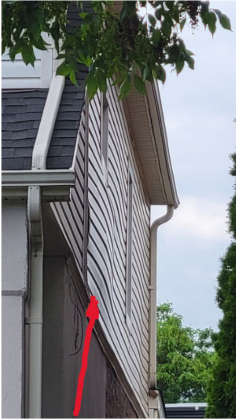
Siding is detached on the north side of the house.
