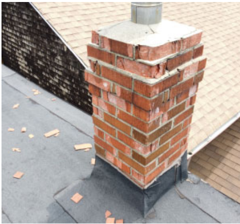
Obsolete chimney- bricks are spalling. repair or remove
