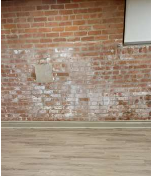
Efflorescence and foundation adjacent to where downspout discharges into the drain/weepers
